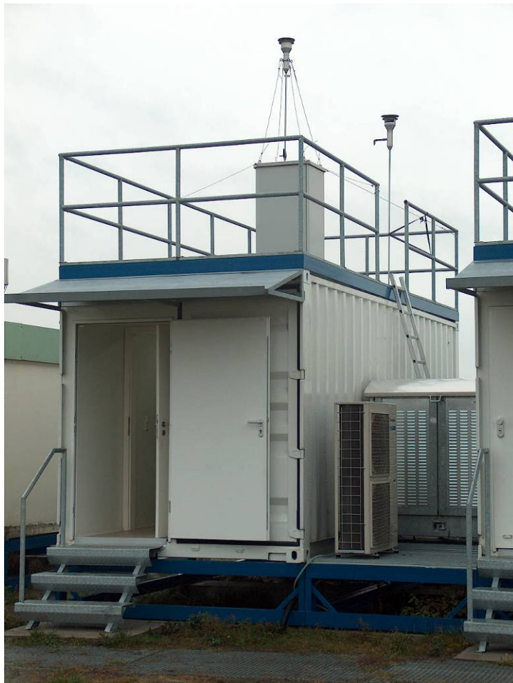
Figure 2: Outside view of the measurements station
